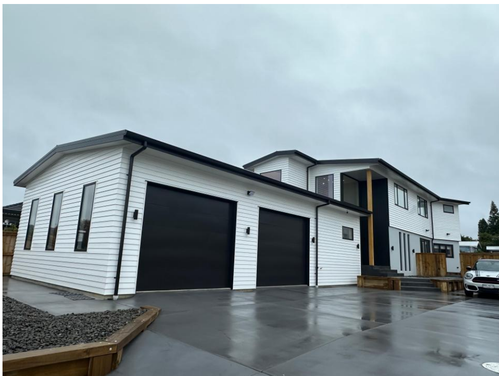
COMPLETED — low-maintenance Palliside® weatherboard cladding on a completed Tauranga re clad
